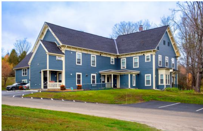
The Farmhouse at Burkeland Lane provides housing to seniors, all of whom were temporarily relocated during renovations.
