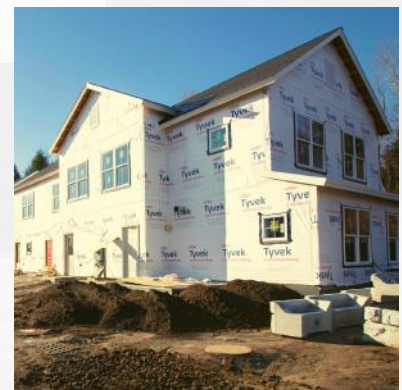
Progress on the new eight-unit building at Burkeland Lane.
