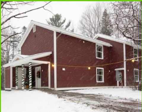
One of the newly-renovated duplexes at Burkeland Lane.
