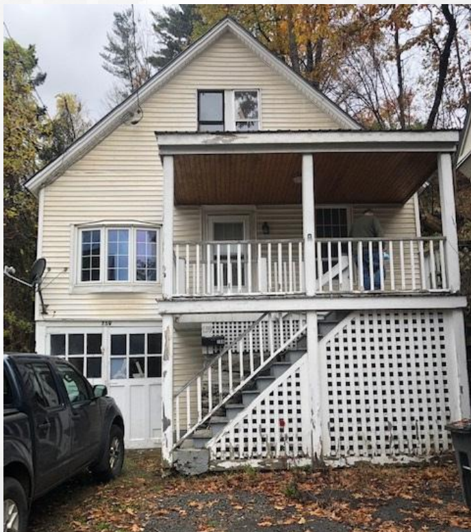
759 Railroad Street, St. Johnsbury
